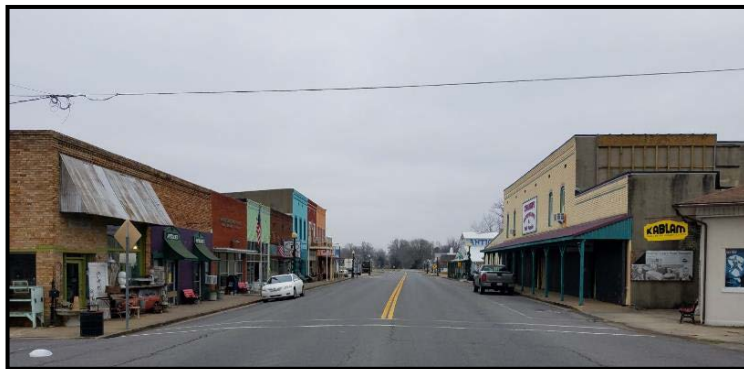
Figure 38: Main Street (US 641) Looking North at Center Street Intersection
