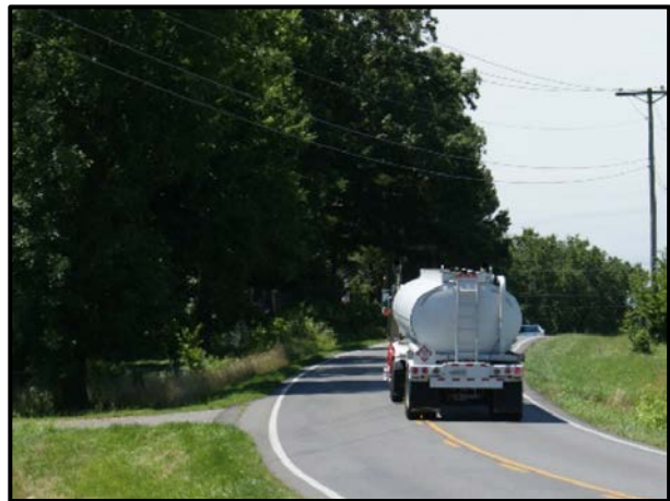
Figure 6: Narrow Lanes and Poor Geometry Create Unsafe Conditions
